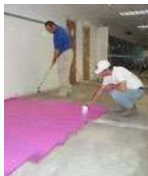
Checking thickness with a wet film gauge
