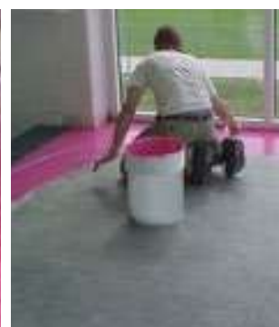
Cut in with trowel or roller to avoid taping
